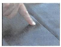
**Step 4**- Test the primer flash-off by touching the primed area with your finger and pushing forward at an angle. The primer should not string as your finger is moved up and away.
