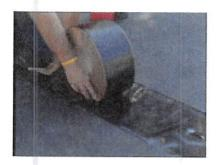
**Step 5**- Install the QuickSeam Cover Strip by using both thumbs in the core and rolling the tape away from your body. As you move forward, peel away the release paper and place it under your knee.
